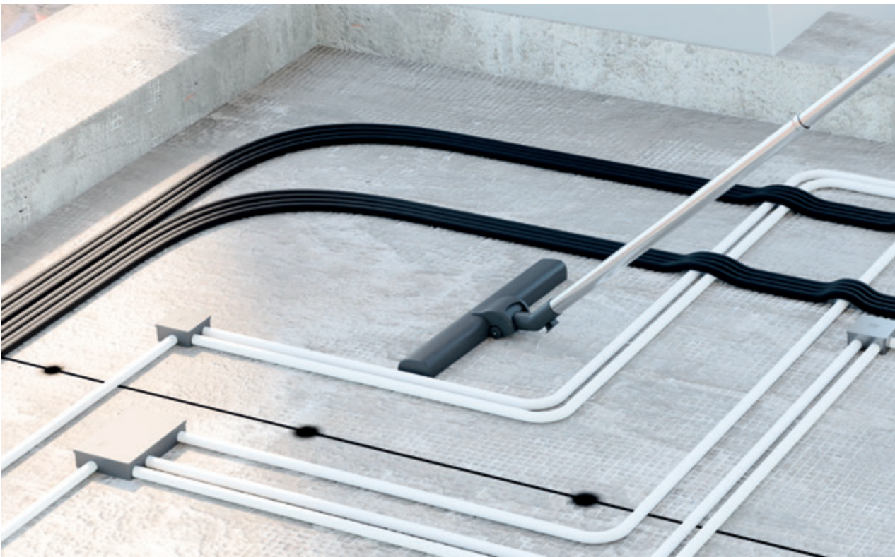
Thorough slab cleaning and suction
