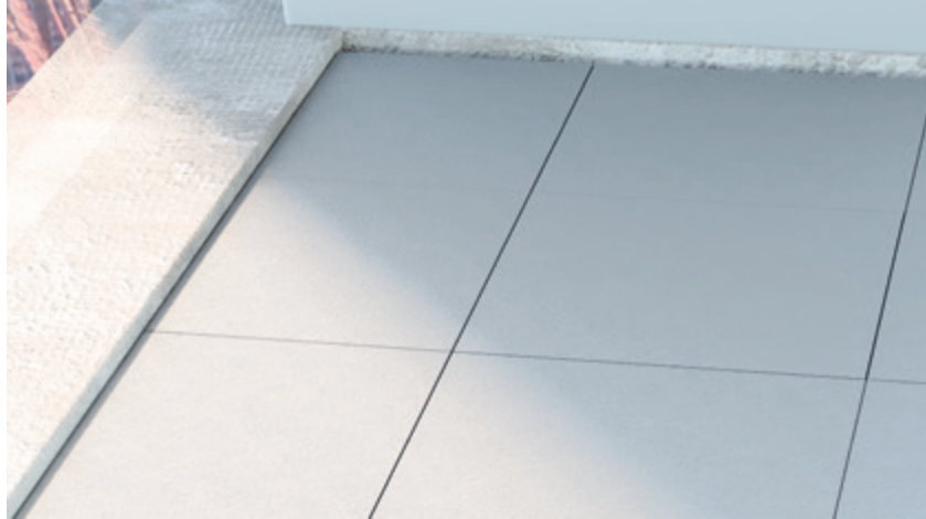
Aligned and levelled panel positioning
