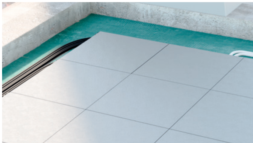
Aligned and levelled panel positioning
