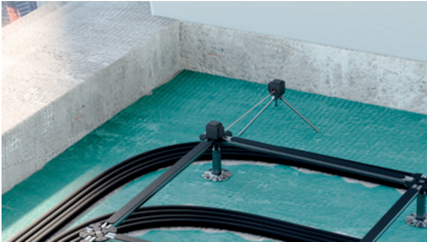
Use of spirit level for positioning posts
