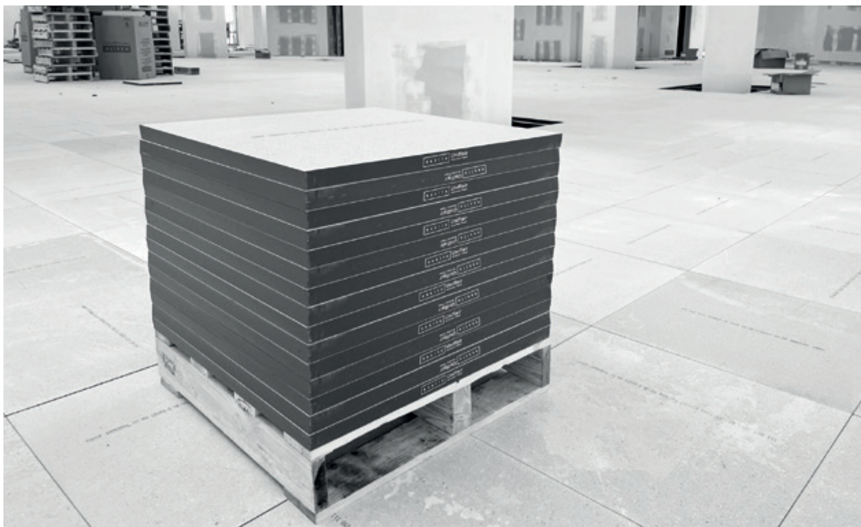
Site conditions. Place component packages only near the installation area
