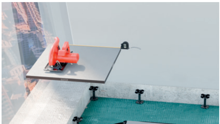
Perimeter panel cutting
