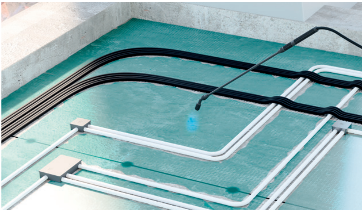
Applying dustproof paint
