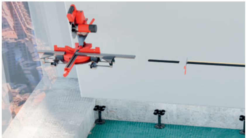
Cutting stringers and perimeter seals
