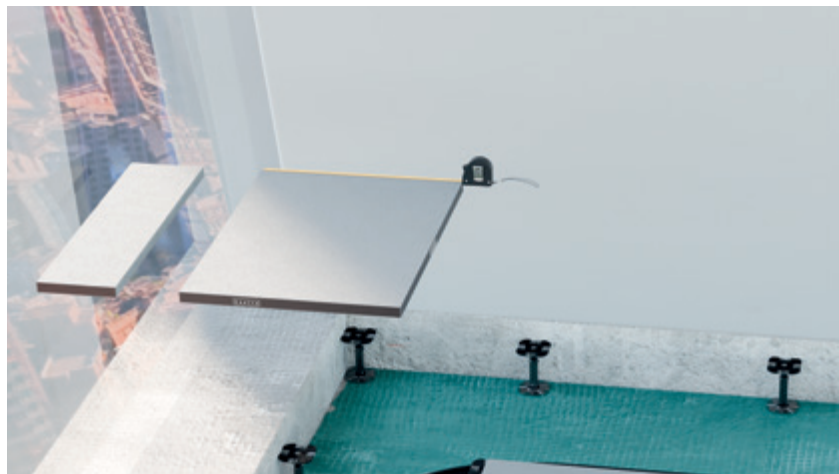
Measuring and cutting perimeter panels
