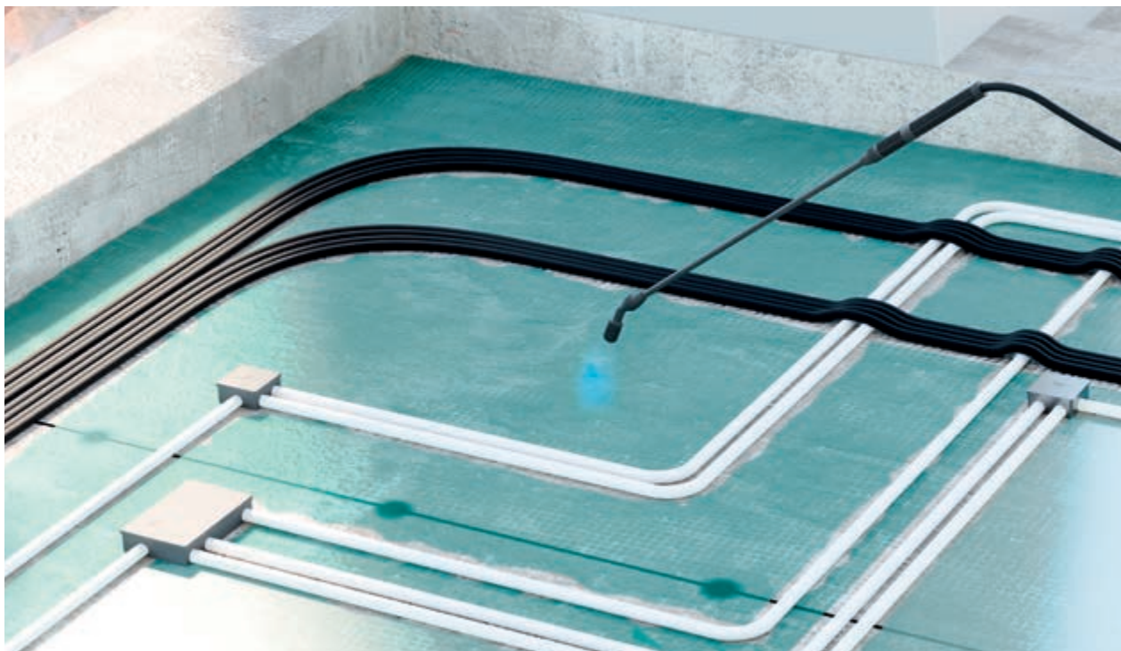
Applying dustproof paint
