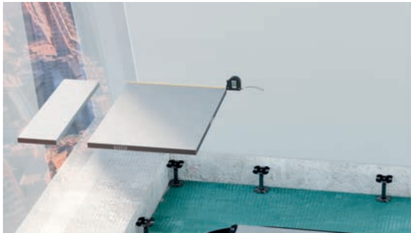
Measuring and cutting perimeter panels
