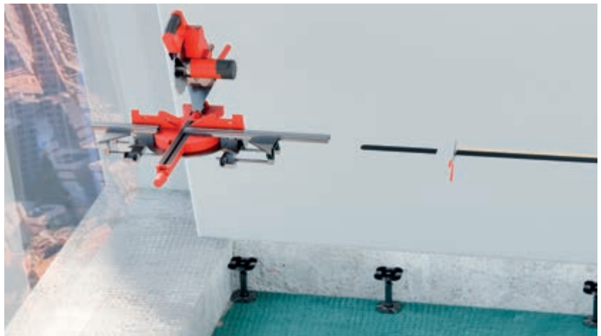
Cutting stringers and perimeter seals
