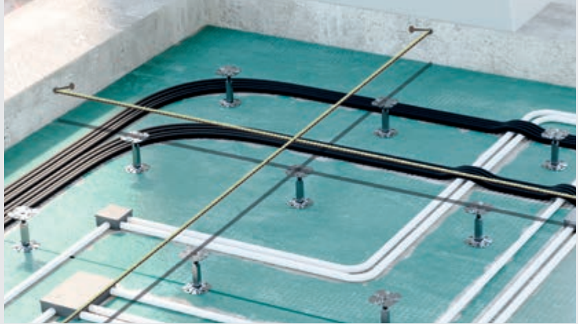
Alignment using the two orthogonal wires
