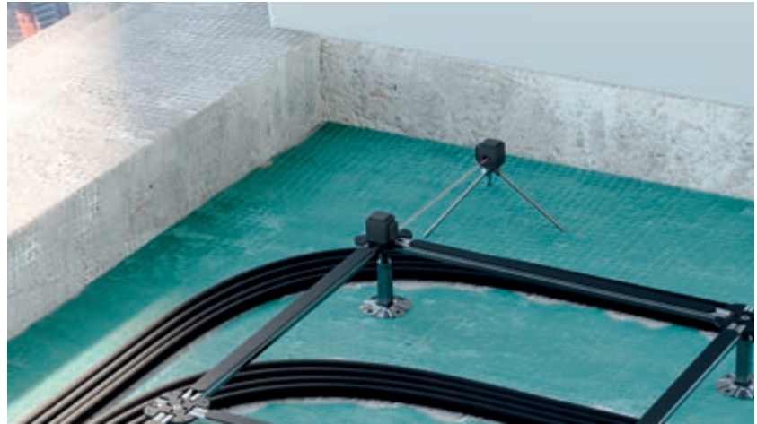
Use of spirit level for positioning posts
