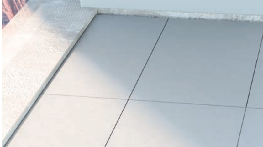
Aligned and levelled panel positioning
