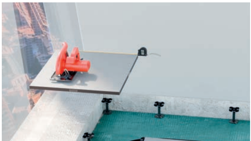
Perimeter panel cutting
