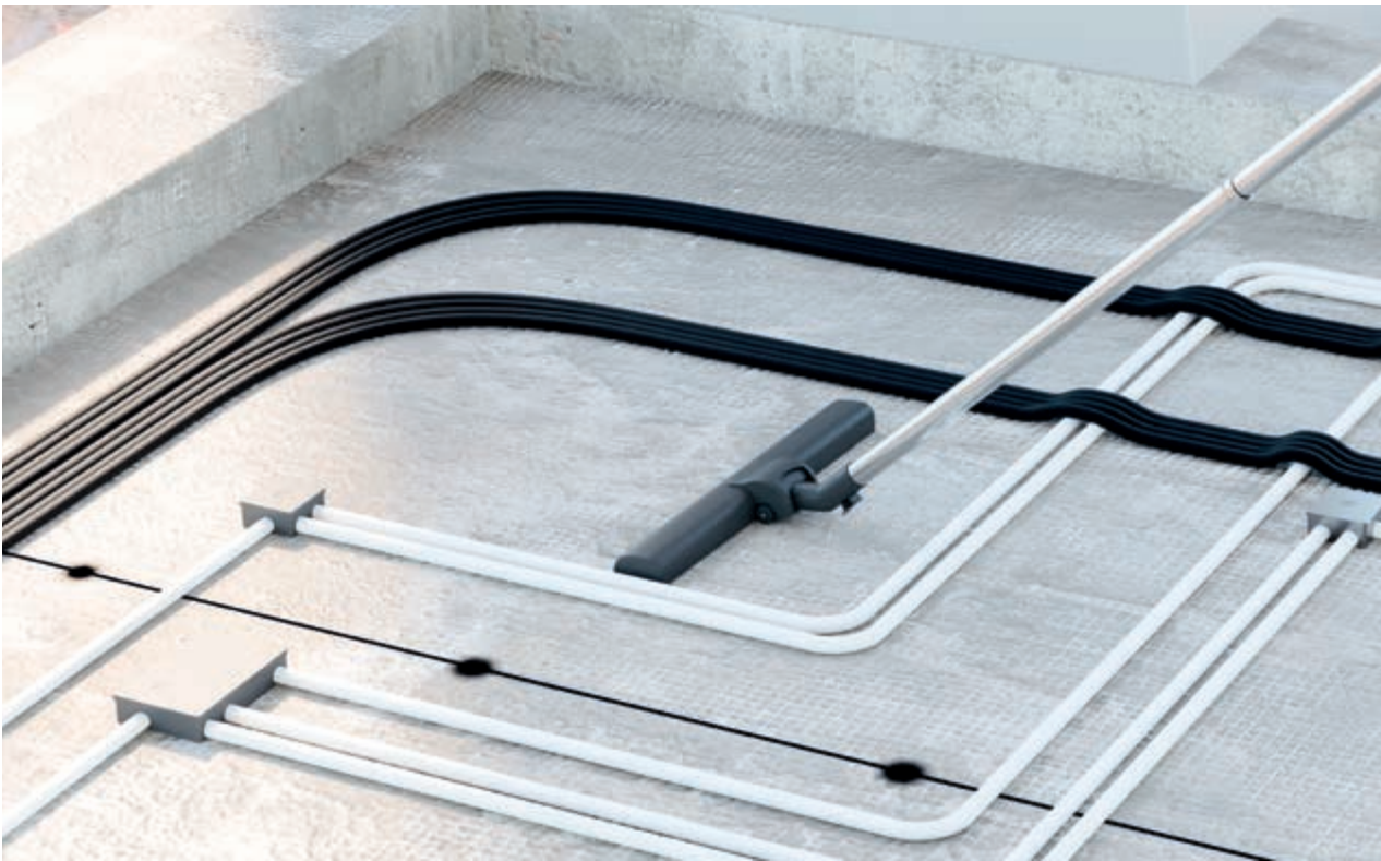
Thorough slab cleaning and suction
