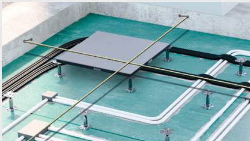
Positioning the first panel using the two orthogonal wires
