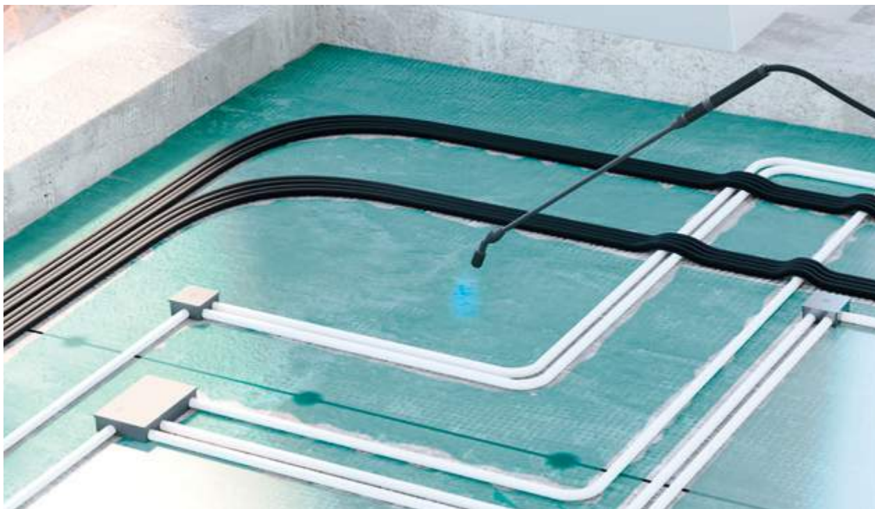
Applying dustproof paint
