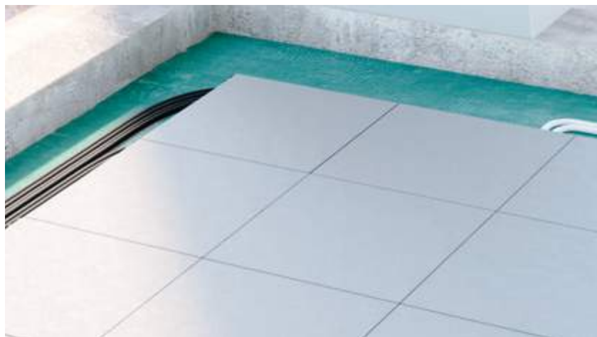
Aligned and levelled panel positioning
