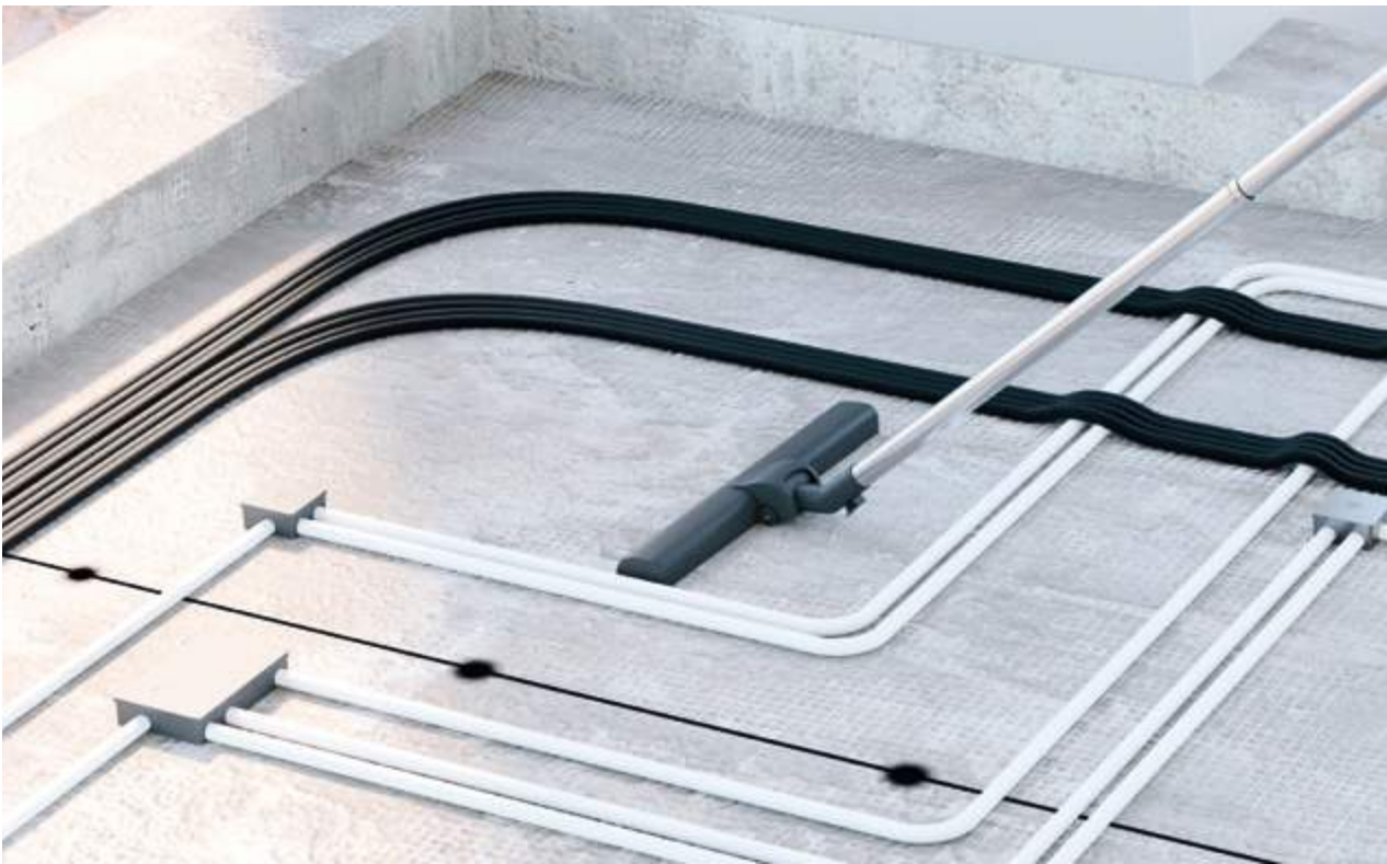
Thorough slab cleaning and suction
