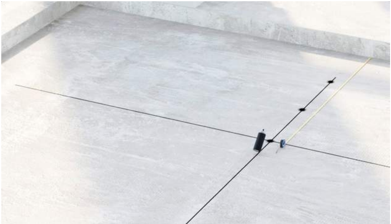
Spray canister marking
