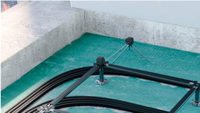
Use of spirit level for positioning posts
