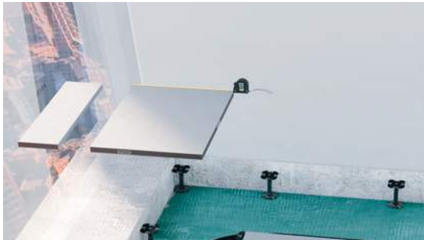
Measuring and cutting perimeter panels
