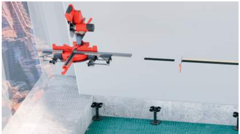
Cutting stringers and perimeter seals
