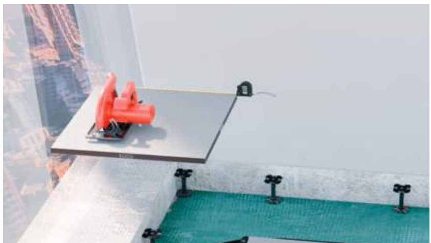
Perimeter panel cutting
