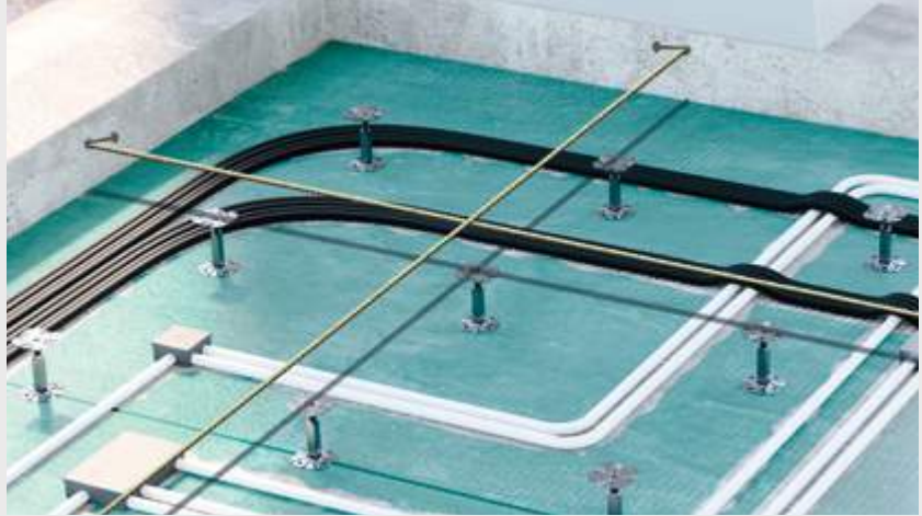
Alignment using the two orthogonal wires
